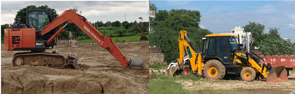
Fig 2.6 (a): Tracked excavator
